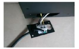
2. Attach the wiring to the junction block. Please make sure the live wire goes into the "L", the neutral wire into "N" and the ground wire into "G".
