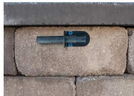
Figure 6.4 – Fasten down the bracket
