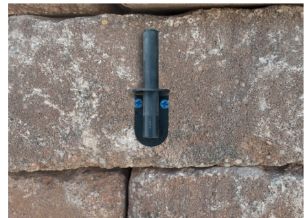
Figure 6.8 – Fasten down the bracket
