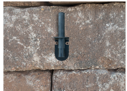
Figure 6.7 – Dry fit the bracket
