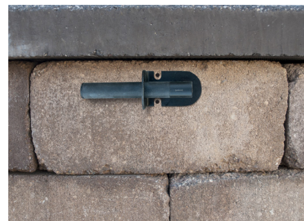
Figure 6.3 – Dry fit the bracket
