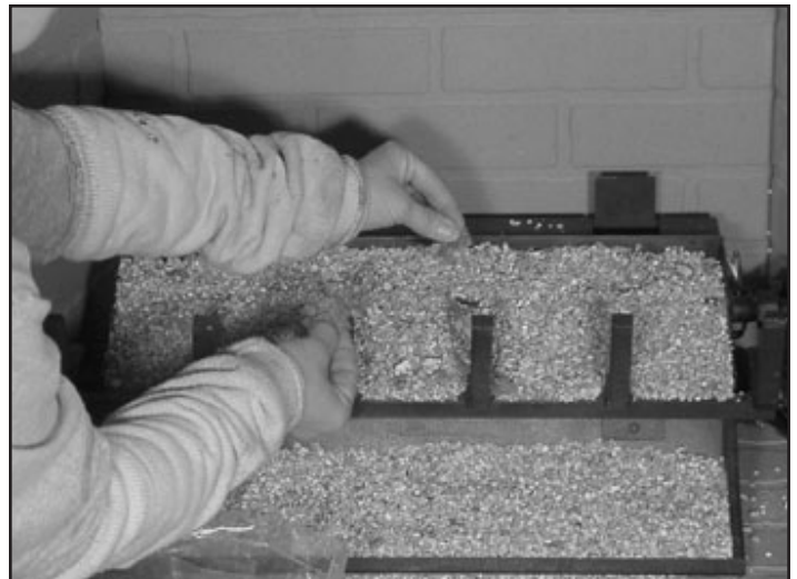
Figure 7 Placing Rock Wool
