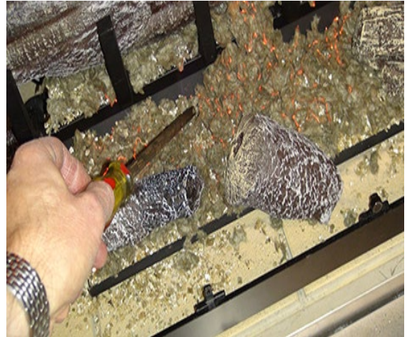
Figure 9- Adjusting of Flame Pattern
