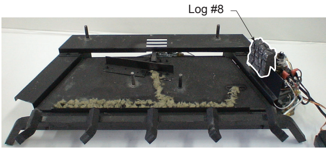
Figure 5.3 - Log #8 Placement
