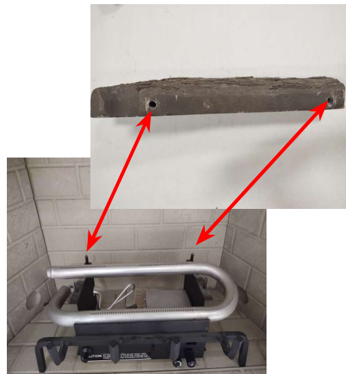
Figure A - Rear Log Placement
