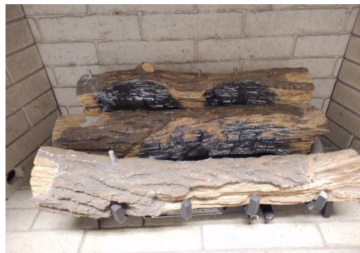
Figure T - Install Front Log
