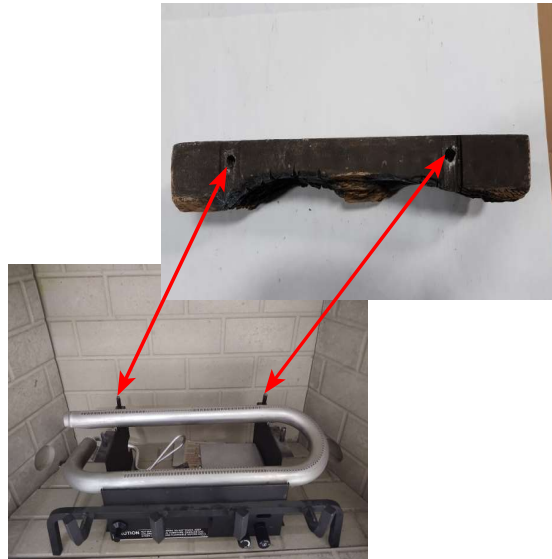
Figure N - Rear Log Placement
