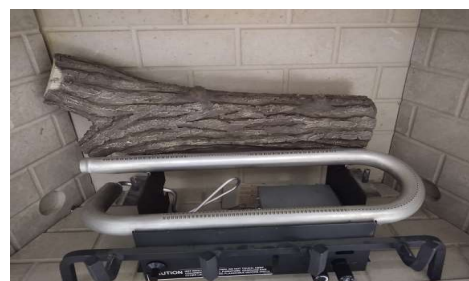
Figure B - Install Rear Log
