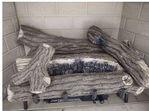
Figure K - Install Top Left Log
