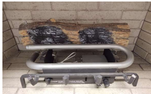
Figure P - Install Rear Log
