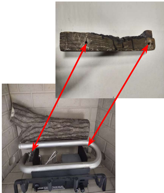
Figure C - Middle Log Placement
