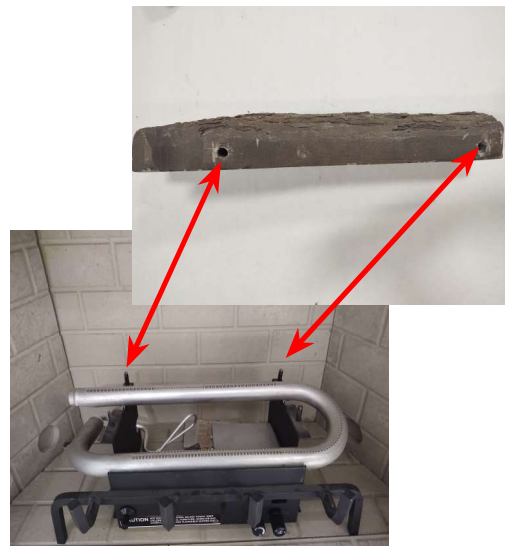
Figure A - Rear Log Placement
